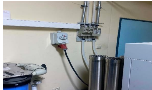
Figure 2: Post-treatment water sampling point in the dialysis unit
